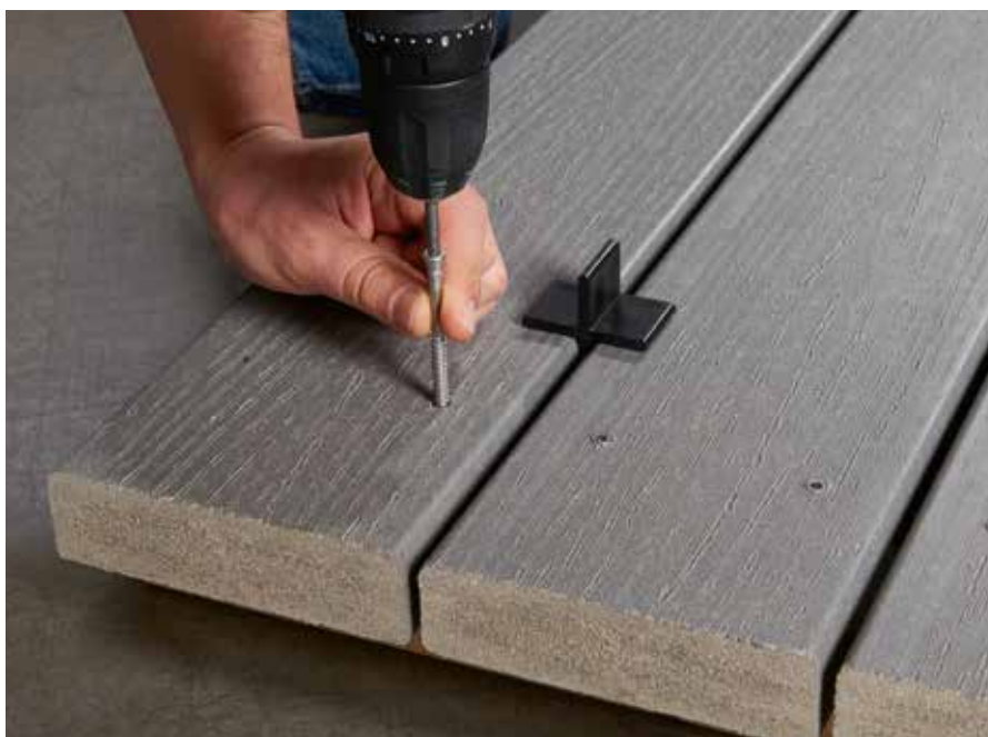
Mounting the load-bearing deck
