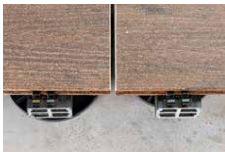
Deck longitudinal joint
